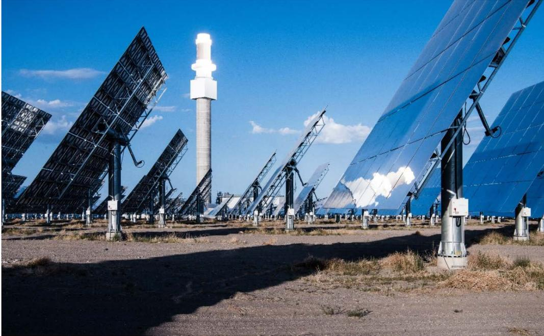
**Figure 2. Power tower concentrating solar-thermal power systems such as this one use focused mirrors, called heliostats, to reflect sunlight onto a receiver on top of a tower. Each heliostat uses a two-axis tracking system to focus the sun on the power tower receiver.**
